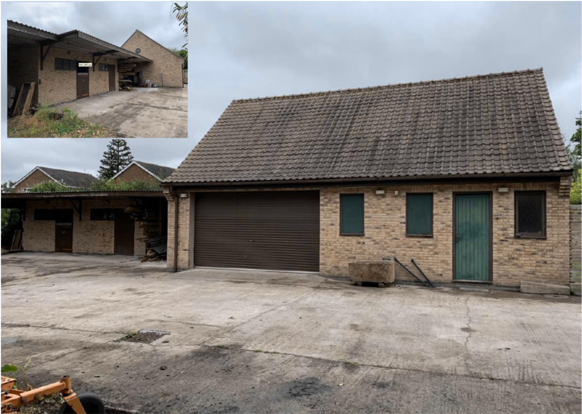
View north of the existing building to be converted
