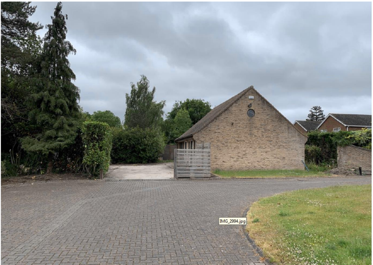
View west of the existing building to be converted
